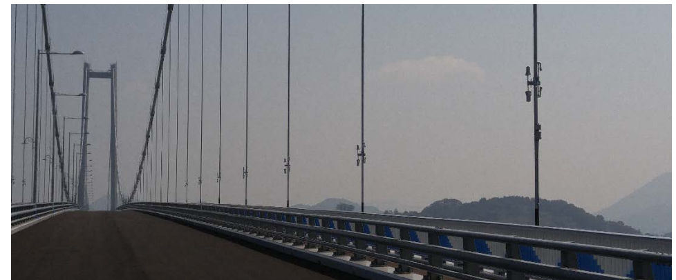
Stockbridge Damper, Palyung Bridge(^ bridge), 2016
