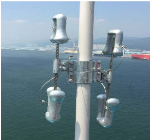
Stockbridge Damper, Ulsan Bridge(suspension bridge), 2015
